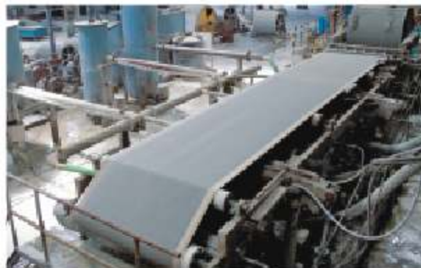
Everest Fibre Cement Boards Plant at Lakhmapur
