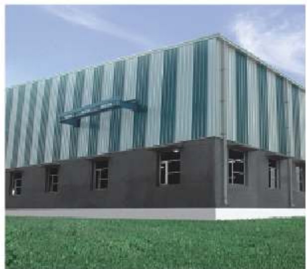
PEB Factory Building
